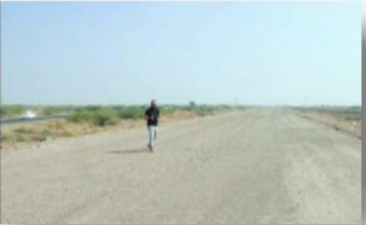
6 LANE EXPRESS HIGHWAY AHMEDABAD-DHOLERA
