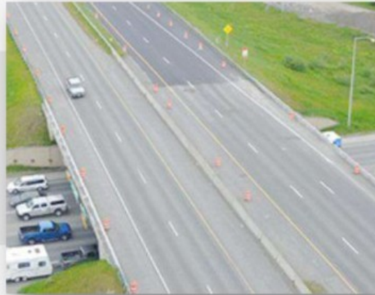
6 Lane Express Highway Ahmedabad - Dholera
